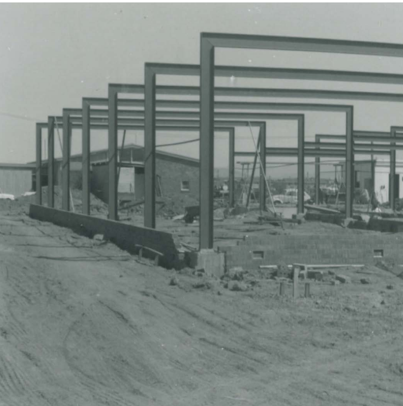
Canberra Tradesmen's Union Club under construction 1964
